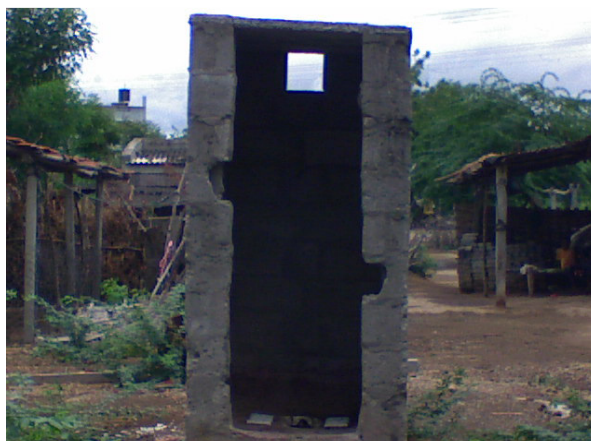
Abandoned ILCS unit at Tumkur, Karnataka
